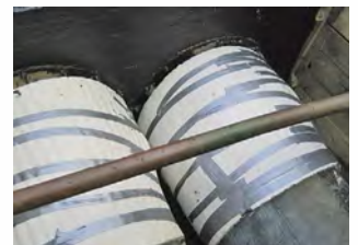
before backfilling protect sealing sleeves with expansion pad
