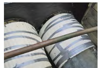
before backfilling protect sealing sleeves with expansion pad
